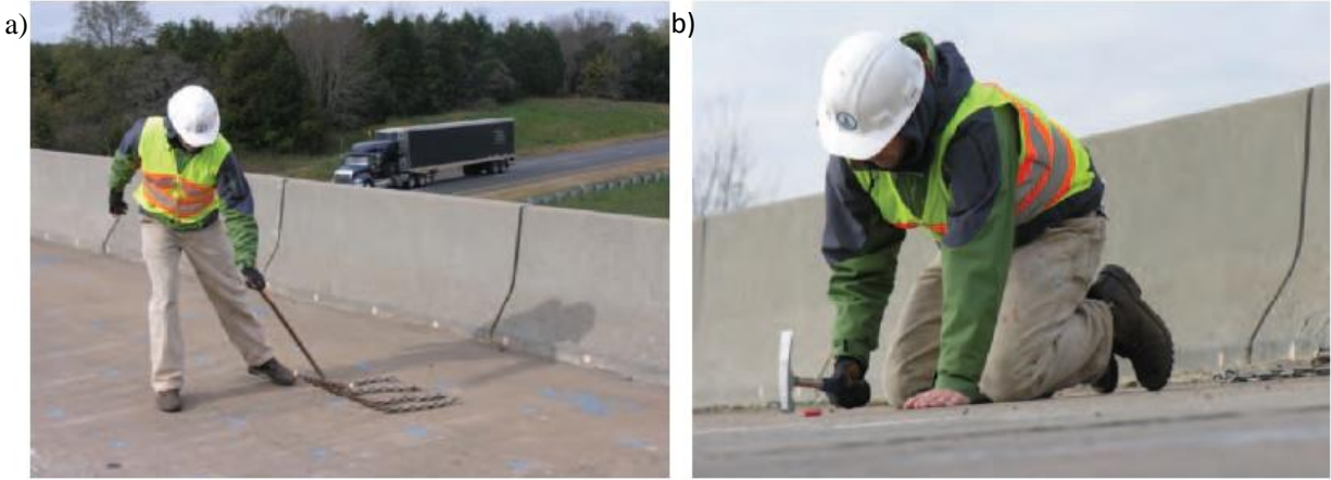
Figure 2-1. a) Chain dragging method and b) Hammer sounding method (Gucunski 2013. Used with permission).
